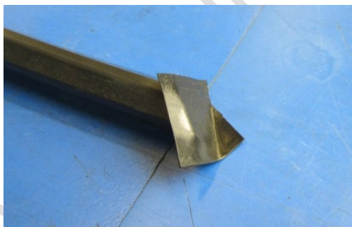
Applying rubber sheet
